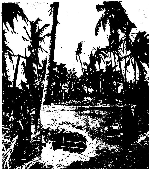
Figure 109. Concrete pillbox on Guam.
